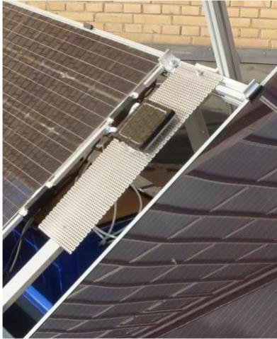
**Figure 15:** Installation of the integrated CuInGaSe -alkaline electrolyser module into the demonstrator test field.
