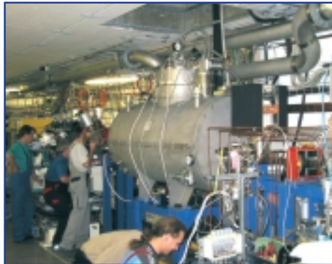
Fig. 1: Installation of the 7 Tesla wavelength shifter for the protein structure factory.
