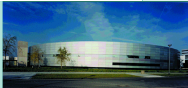
BESSY storage ring facility
