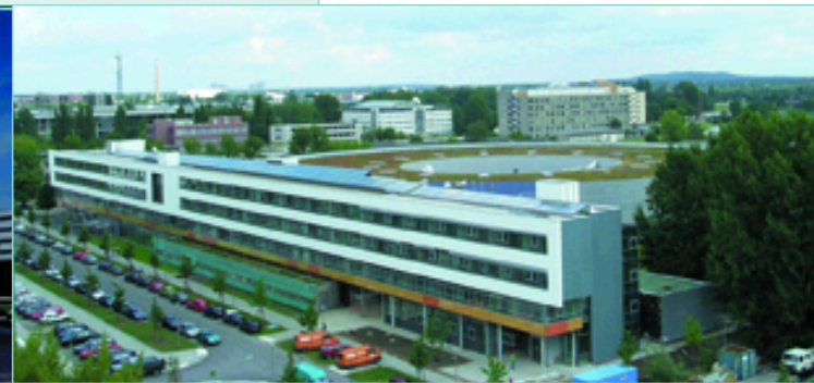
Office and laboratory building
